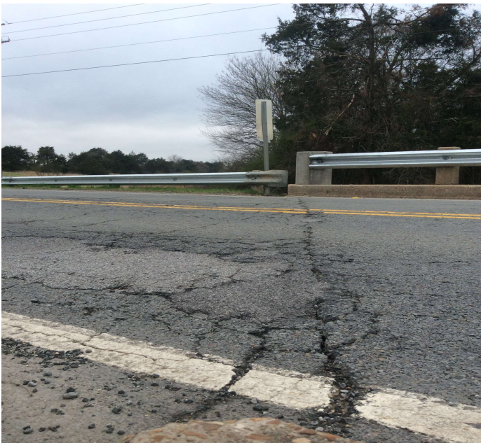
PHOTO 1 Description Visible settlement to Roadway @ Abutment 1 & 2.
