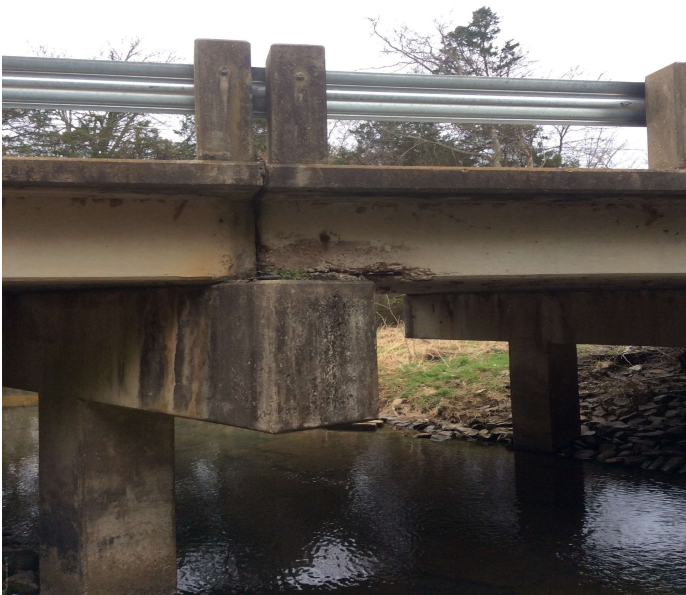
PHOTO 1 Description Spall with 1' rebar exposed to outside edge of deck on Right side of Span 2.
