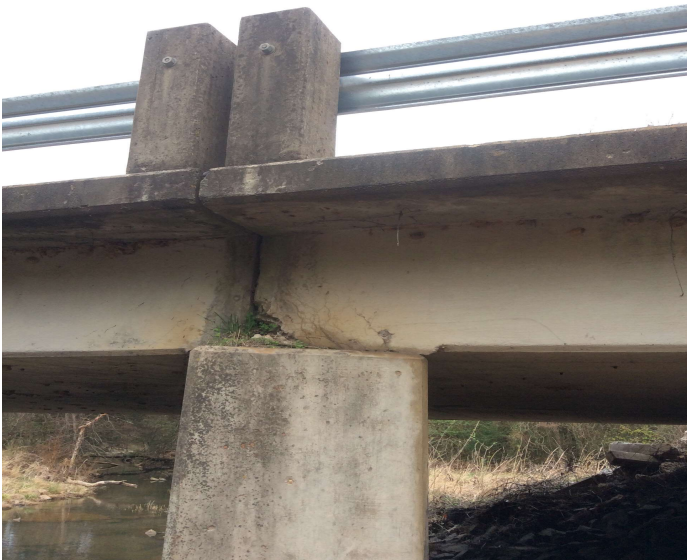
PHOTO 1 Description Cracks to outside edge of deck over Bents 1 & 2.
