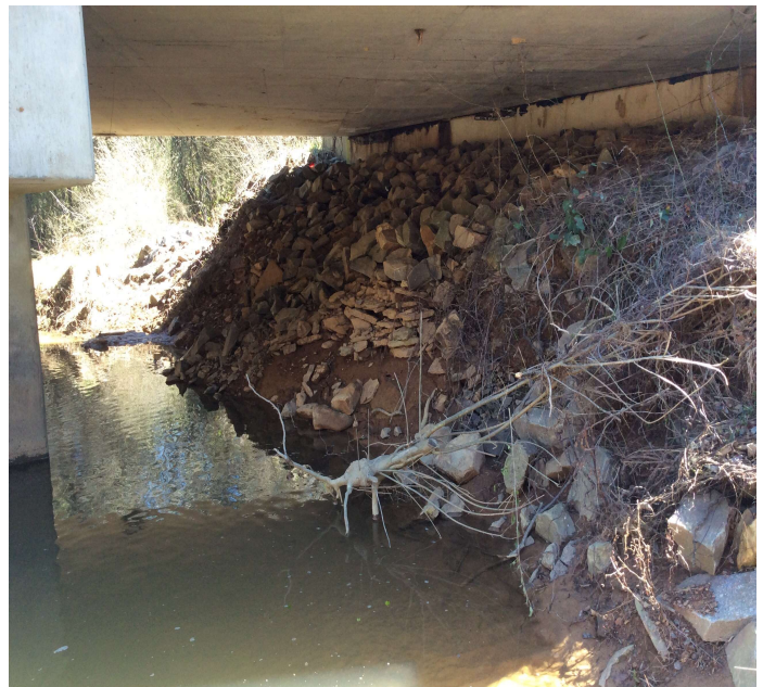
PHOTO 2 Description Severe erosion to Slope @ Abutment 1.
