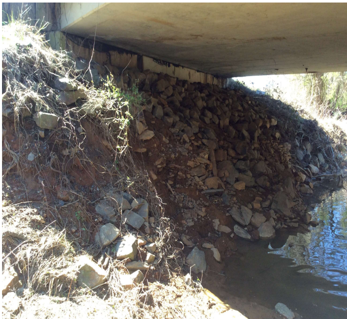
PHOTO 1 Description Severe erosion to Slope @ Abutment 1.
